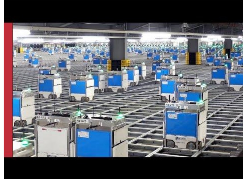
Ocado, London, grocery warehouse.
