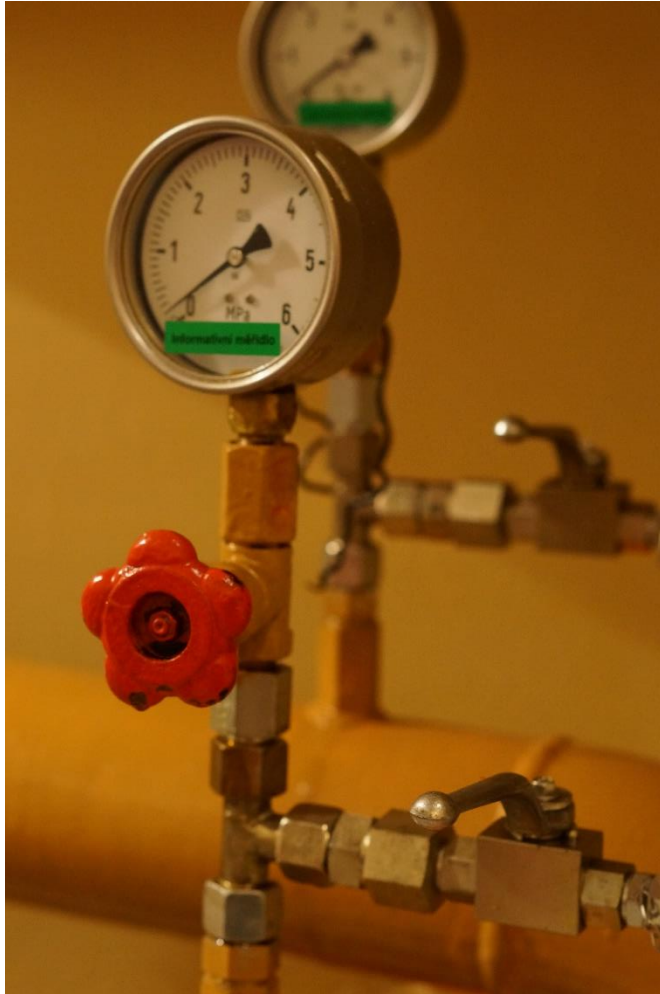
Hydroelectric power station Orlik
