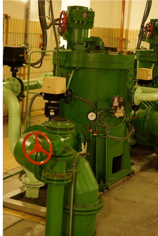
Hydroelectric power station Orlik
