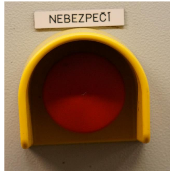
Hydroelectric power station Orlik
